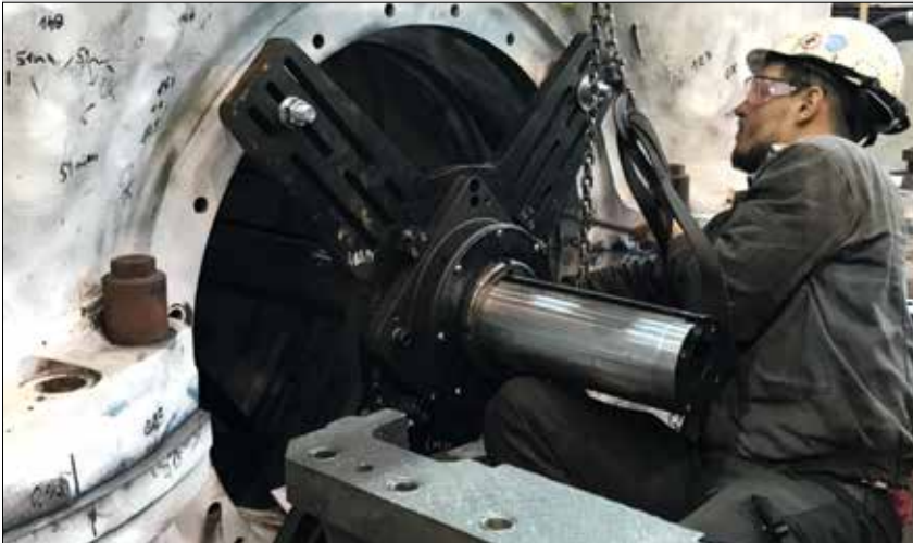
▲ Pipe cutters and weld preparation.
